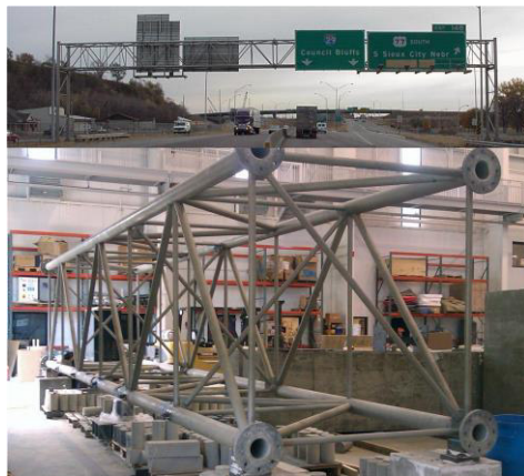
Figure 1 The sign support structure over Interstate I-29 when it was in service, and in Bowen Lab, Purdue University
