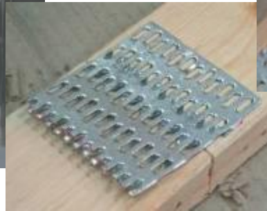
Tooth plate connections
